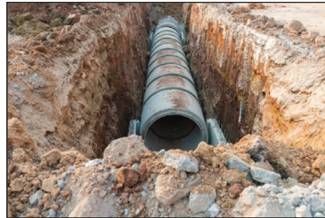
Laying new surface water sewers / upsizing existing
