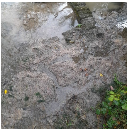
RAG sewage (Image: South West Water)
